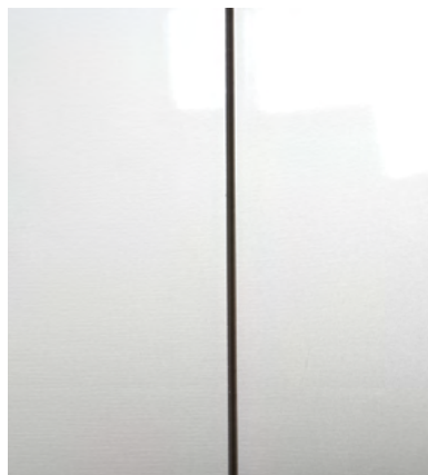
Figure 1: Butt joined sheets prior to application of sealant.
