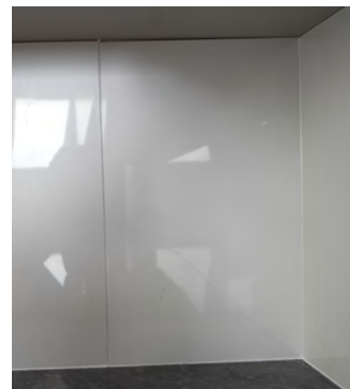
Figure 3: Metaline splashback showing butt join with sealant.
